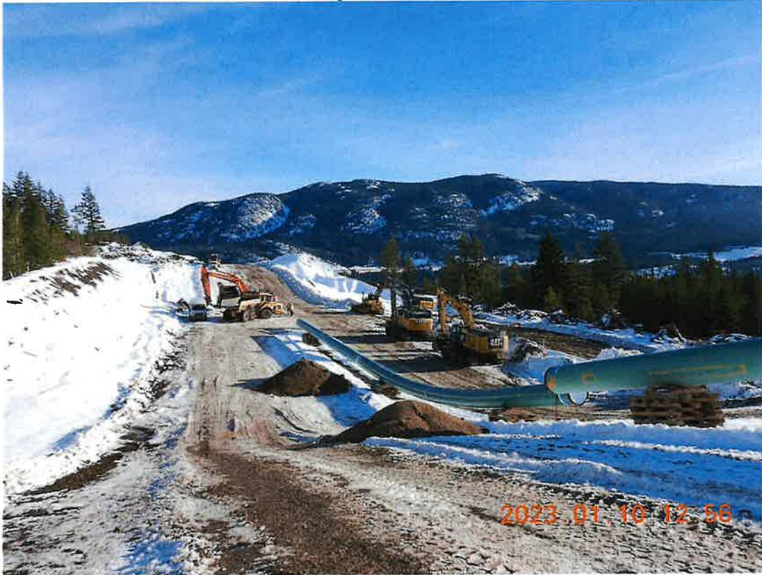
Figure 1 Ditch Bedding
