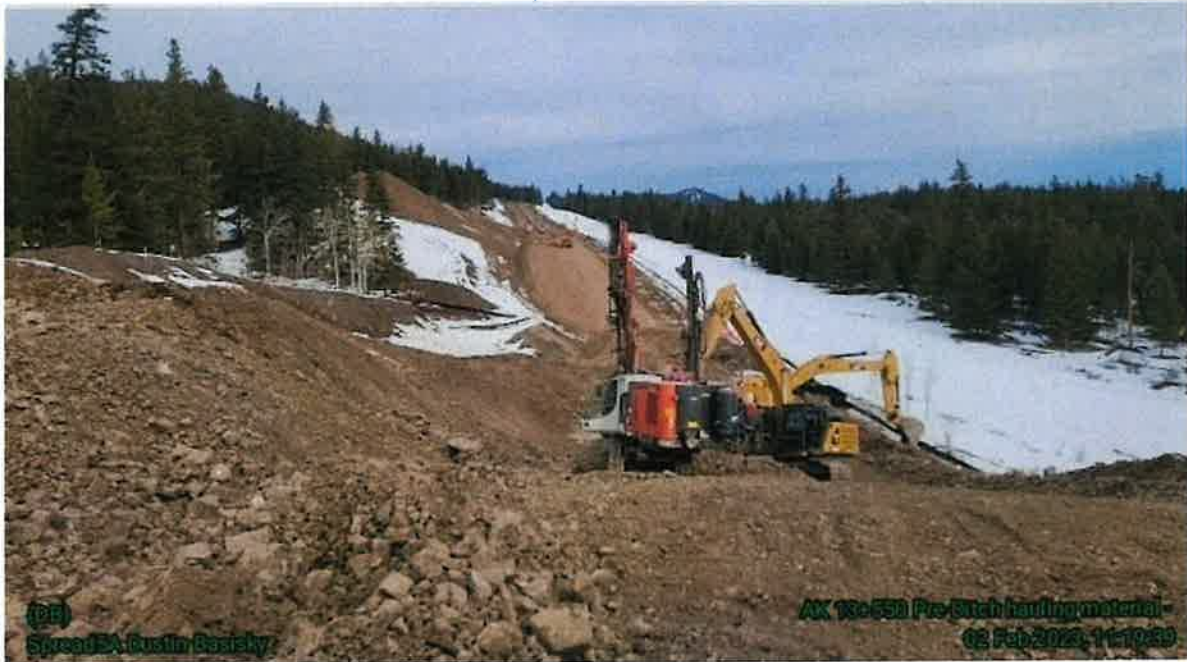
Figure 3 Pre-Ditch Pulling Material on Work Side
